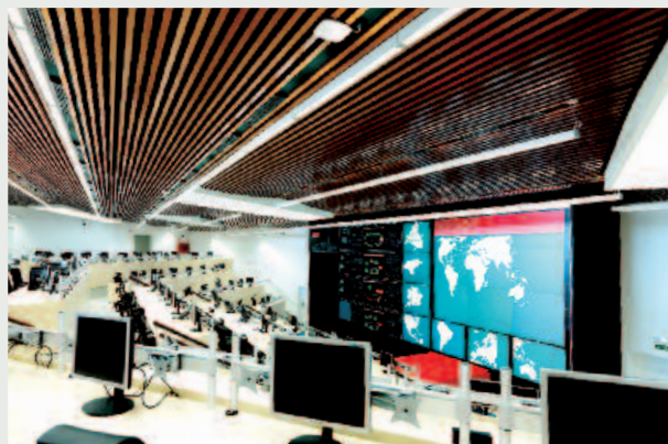
The Group's new data processing centre in Cantabria, Spain
