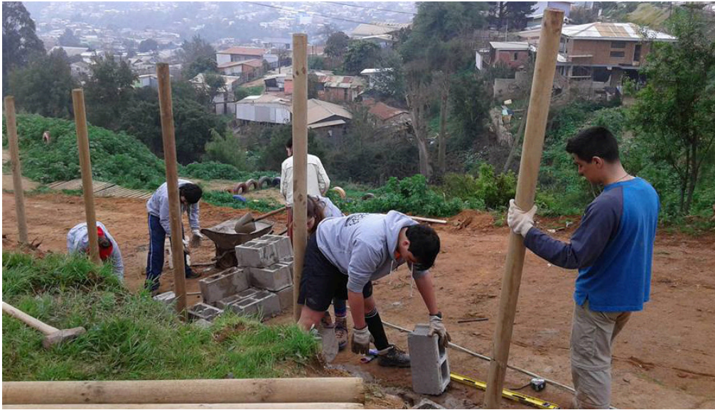
Building homes in partnership with TECHO Chile.
